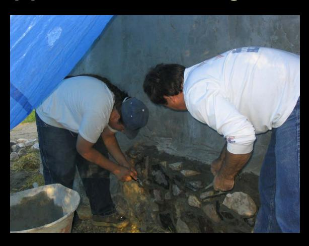
Mix three parts sand to one part clay. Add straw and some manure. Add water till the mixture feels like lumpy oatmeal that is not glossy. Then test it on the straw and check it in a week. It is a good mixture if the mud is still on the wall! Start mudding!
